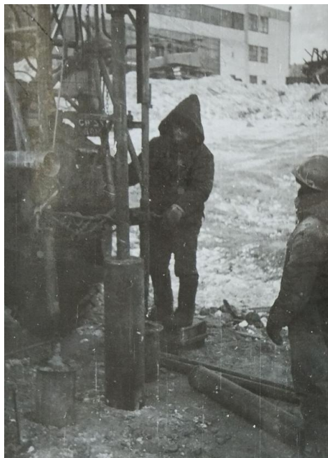
Fig. 2. Shortened core barrel with a diameter of 273 mm (Ulyanov, 2019, 2021)
