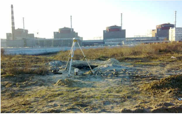
Fig. 2. Well 4602 in the tectonic fault zone of the Zaporizhzhia NPP site before retrofitting
