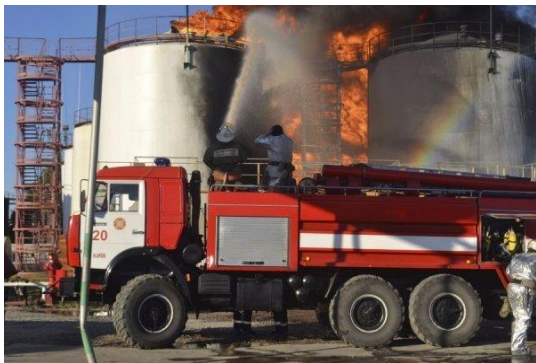
Fig. 1. Fire at an industrial site – formation of a thermal pollution area at an industrial site [ https://www.volynpost.com/news/51948-masshtabna-pozhezha-na-naftobazi-pid-vasytkovym-foto/ ]
